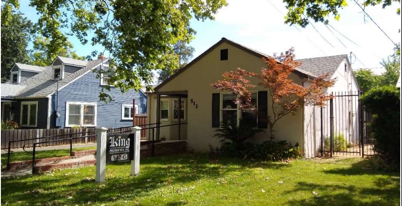
West and south facades, ESA, June 2022
