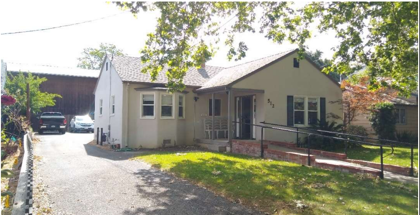
North and west facades, ESA, June 2022
